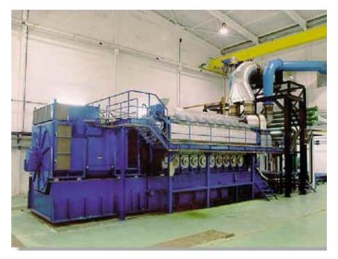
In a synchronous generator, a DC current is applied to the rotor winding producing a rotor magnetic field. The rotor is then turned by external means producing a rotating magnetic field, which induces a 3-phase voltage within the stator winding.
